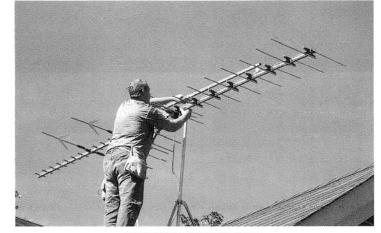
14. The photograph below shows a television antenna being attached to the roof of a house:
